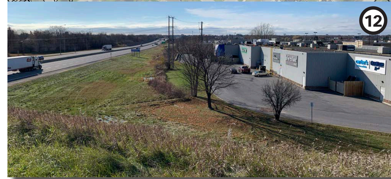
Open area with very limited vegetative screening of adjacent commercial, retail and hospitality land uses.
